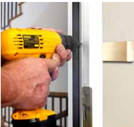
4. Close the door and position the closing jamb so that it makes full and uniform contact with the frame seal. Then fix (as step 3).
