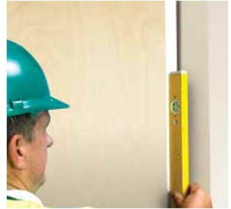
2. Hold the frame in place using wedges, ensuring the frame is square. A large (5ft/1.5m recommended) spirit level should be used to ensure that all jambs are square and plumb.
