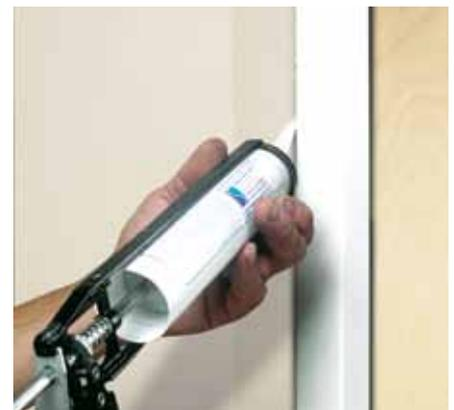
6. Fill the gaps between the frame and wall with a suitable fire resistant infill and sealant capping.
