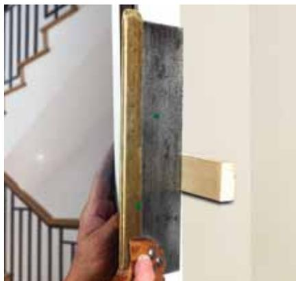
5. Cut off the wedges to align with the edge of the frame. Take care not to damage the surface of the Ecoframe.
